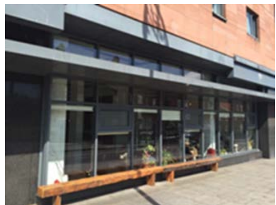
Figure 6: On Street Bench at Fumbally Cafe
